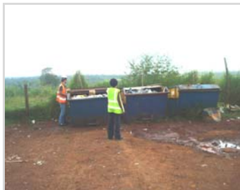
Waste skips for different categories of waste at the dam site
