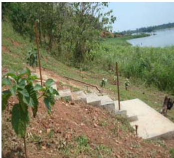
NRE concrete stairway at Namiyagi – Mukono District
