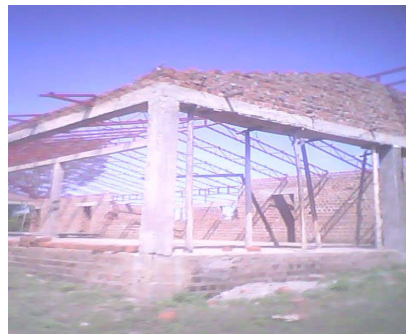
NRE rafting takeout site under construction in Nazigo, Kayunga
